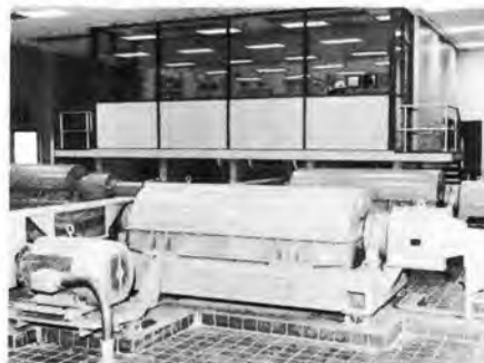
COLUMBIA, S.C. — four P-5400 Super-D-Canter centrifuges used to dewater anaerobically digested sludge prior to incineration.
