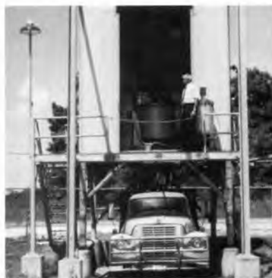
BAYTOWN, TX. — one SludgePak centrifuge dewatering aerobically digested sludge.
