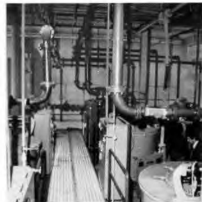
DALTON, GA. — five SludgePak centrifuges dewatering aerobically digested sludge prior to landfill.
