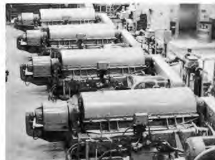
MINNEAPOLIS, MINN. — four P-5400 Super-D-Canter centrifuges used to dewater softening plant sludge.
