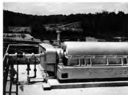
INTRENCHMENT CREEK, ATLANTA, GA. — one P-5400 Super-D-Canter centrifuge used to dewater anaerobically digested sludge for landfill.
