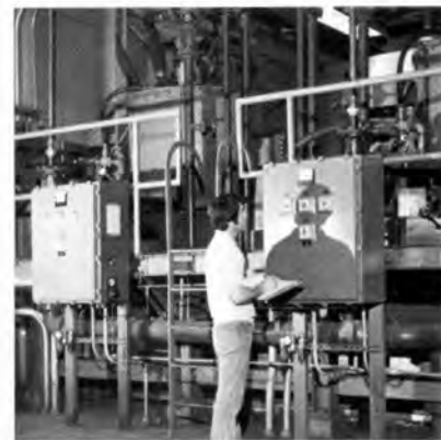
WASHINGTON STEEL, WASHINGTON, PA. — two SludgePak centrifuges dewatering neutralized pickle liquor.
